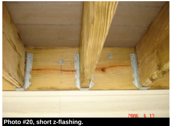
Photo #20, short z-flashing.
