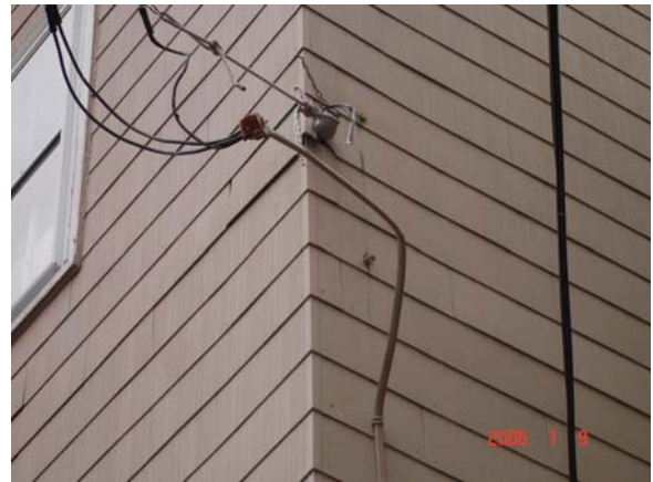
Service secured by rope
