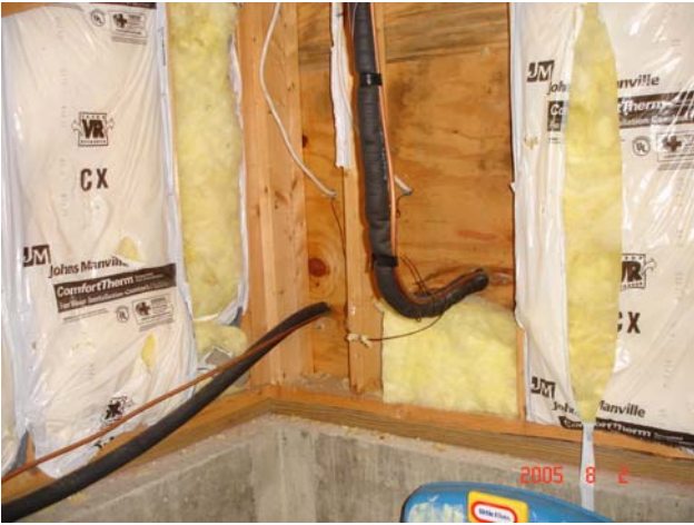
Missing insulation
