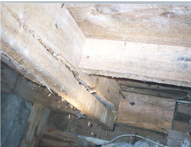
Cracked joist
