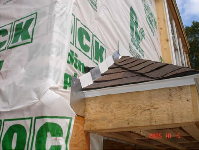
Improper flashing
