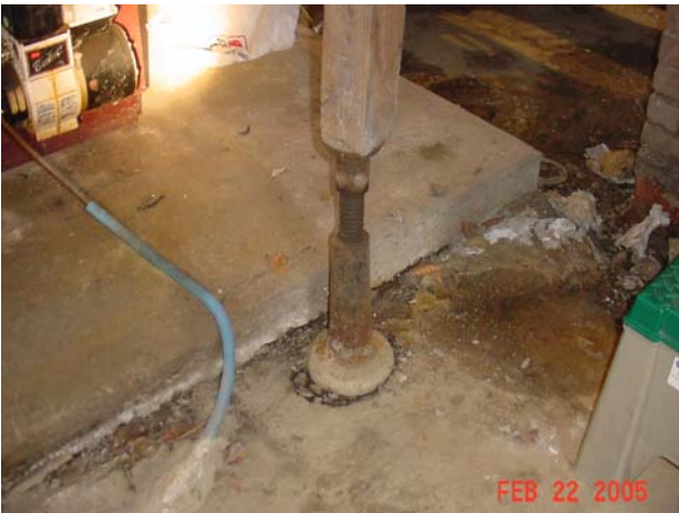
Jack supporting the floor
