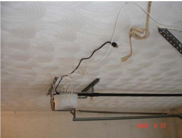
No outlet for door opener
