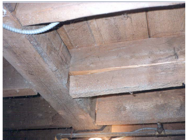
Cracked joist
