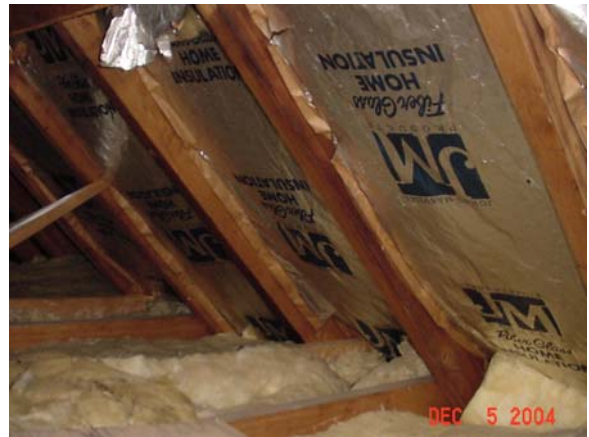
Insulation against roof
