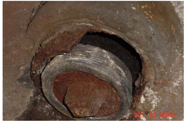
Open sewer line
