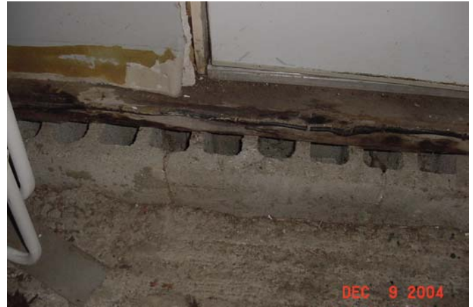
Top cores of blocks not filled
