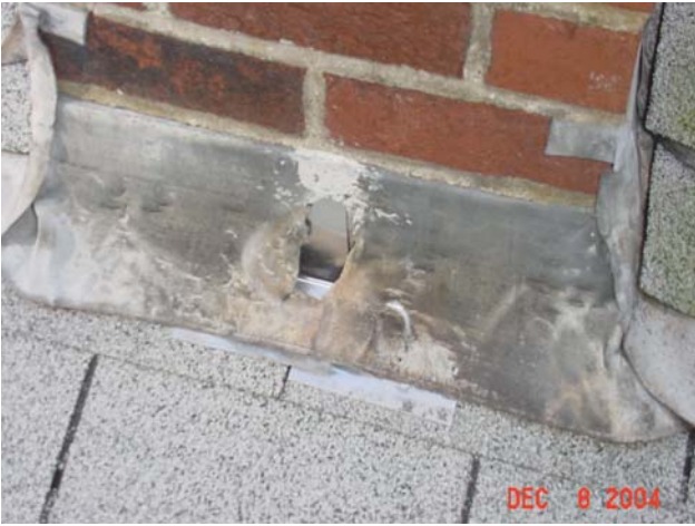
Defective flashing
