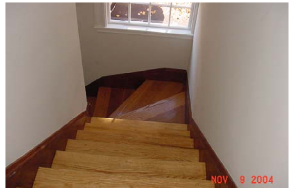
Missing handrail
