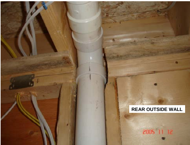
Beware of plumbers!
