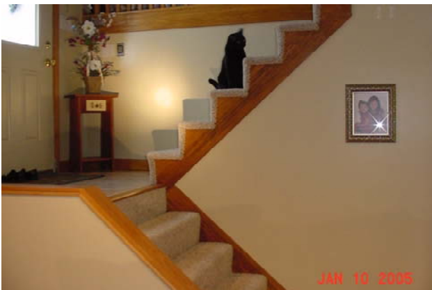
UNSAFE – missing handrails
