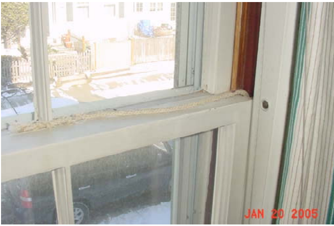
Unsafe, broken sash cord
