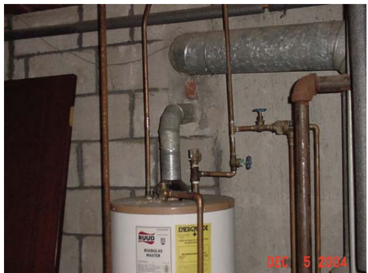
Improper venting
