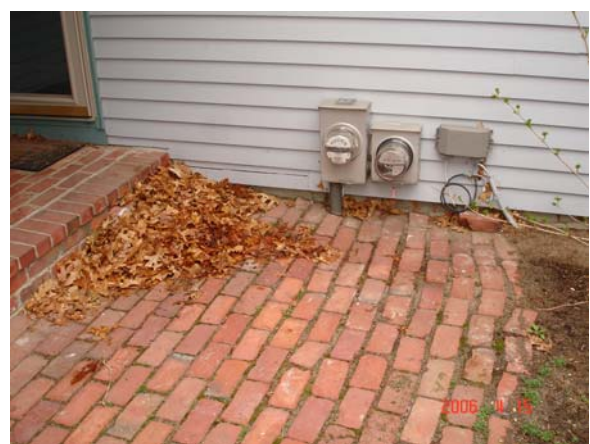
Meters too low
