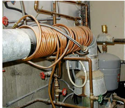
Amateur heat exchanger
