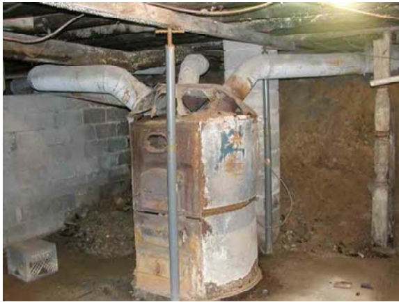
Obsolete gravity furnace
