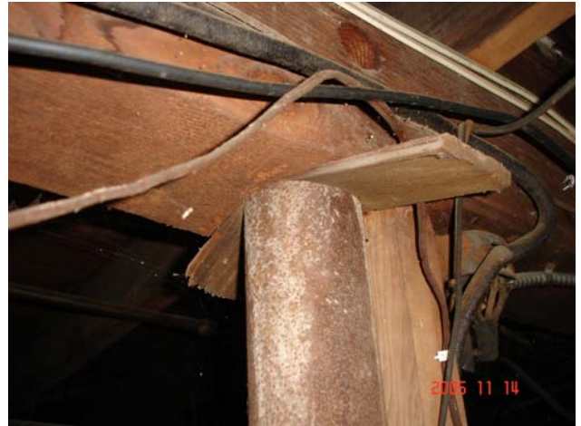
Post compressing into girder
