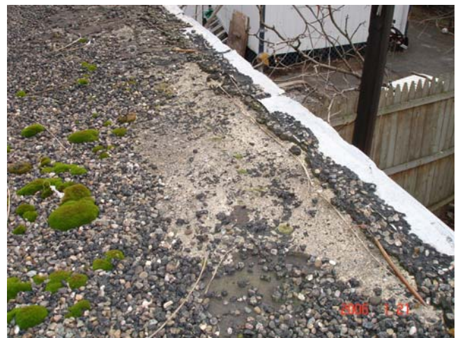
Aged tar & gravel flat roof
