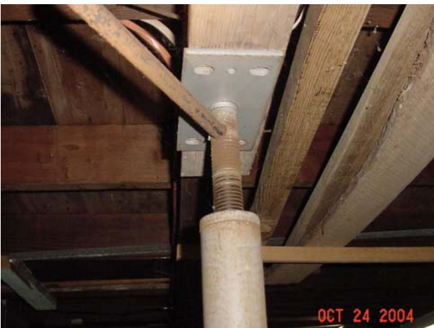
Telescoping columns are for repairs only
