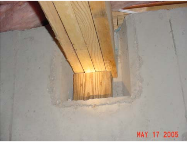
Wood shim supporting girder
