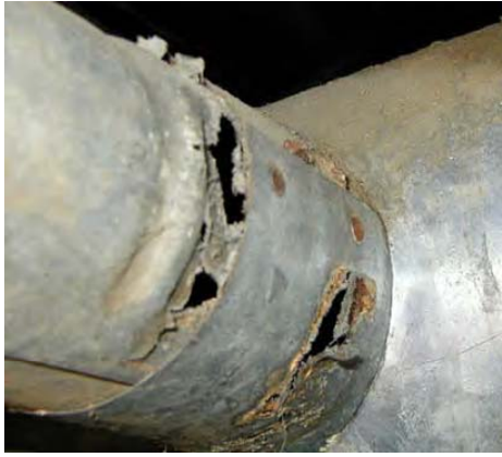
Rusted out flue pipe
