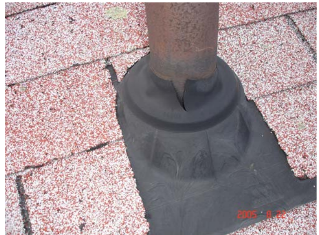
Defective flashing
