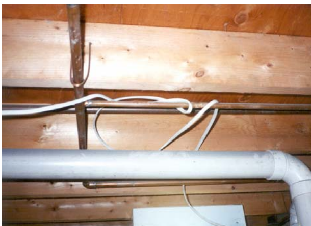
Wired wrapped around pipe
