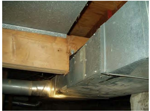
Over-notched joist
